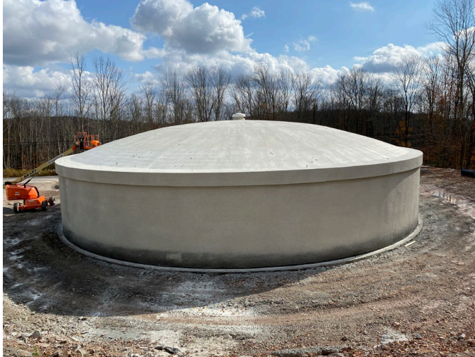
Figure 4. New Route 55 water storage tank
